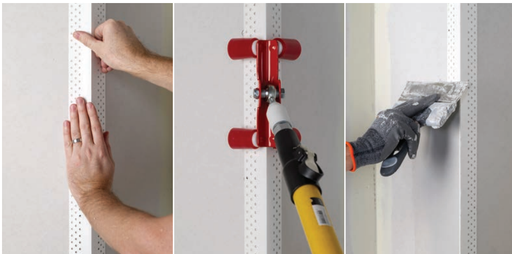
AquaBead is a self-adhesive corner bead with a water-activated adhesive.
