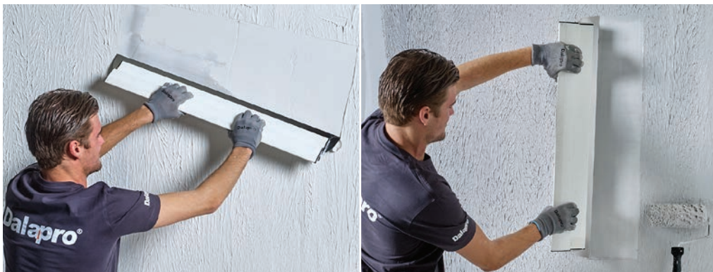
Smoothing the filler after rolling is convenient and easy. Then comes the sanding.
