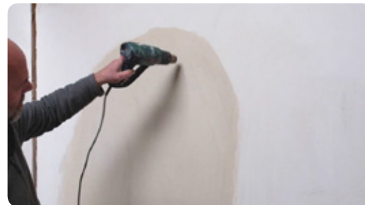
Drying the surface with a heat gun (3:30) ⌚
