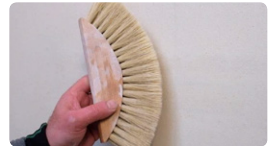
Final phase: brushing the surface (4:30) ▶
