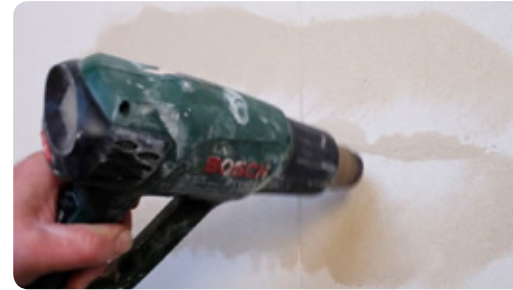
Drying the surface with a heat gun (2:00) ▶
