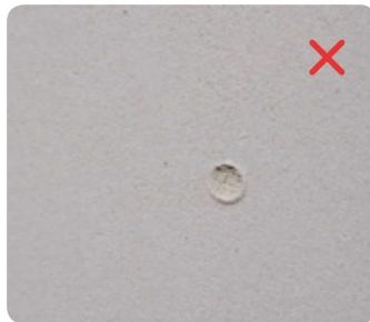
Surface too wet
